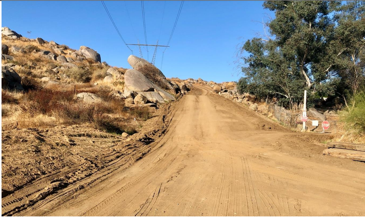
Photo 12 - Access road work between towers 144 and 145. Photo facing west
