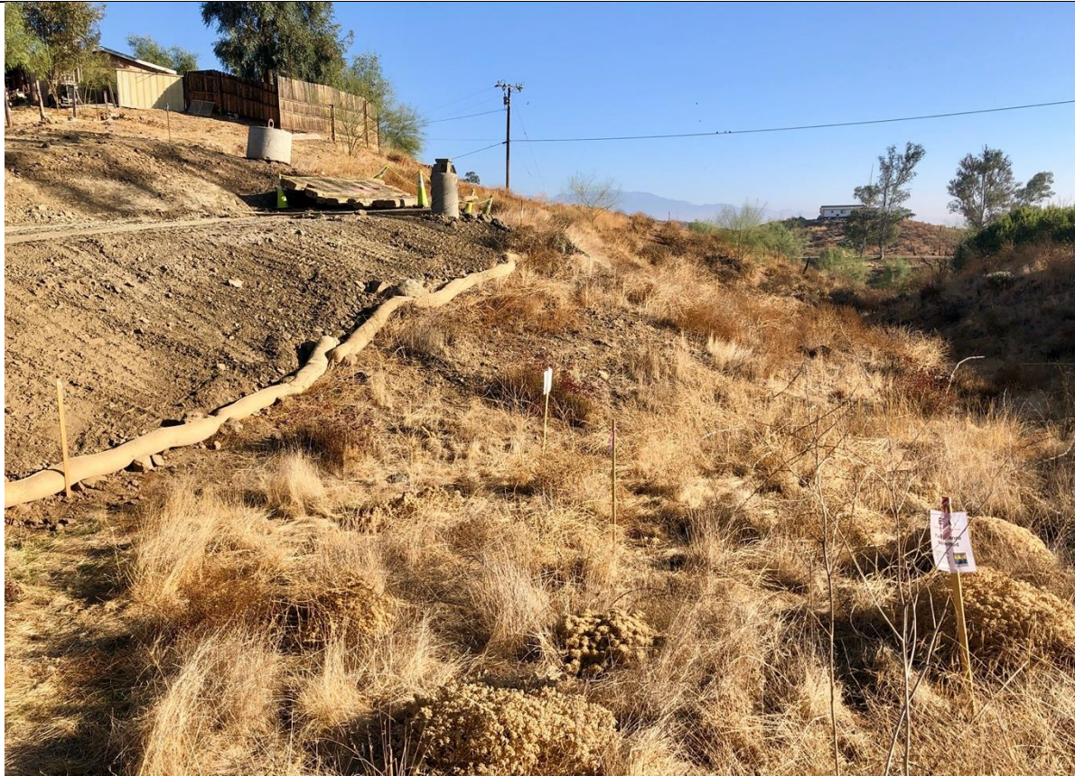
Photo 11 – Tower site 144 with BMPs and ESH signage. Photo facing east
