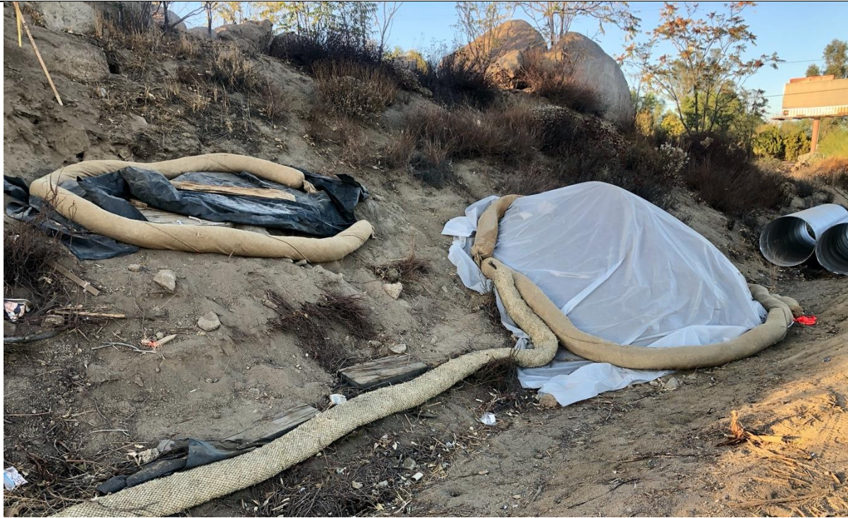
Photo 7 – Foundation work at Pole site 212. Photo facing northeast
