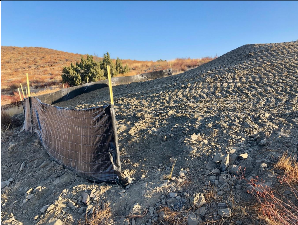
Photo 7 – BMPs for the grading work at tower site 129. Photo facing northeast
