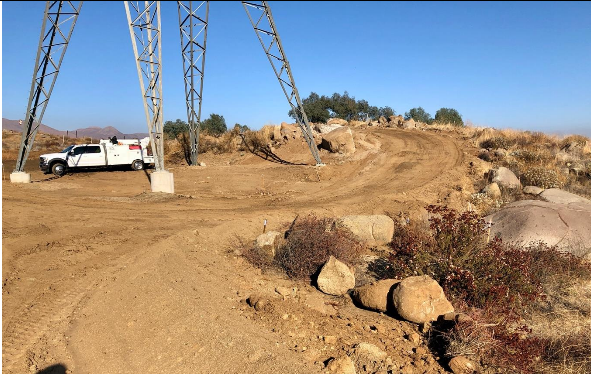
Photo 14 – Access road work around tower site #145. Photo facing northwest
