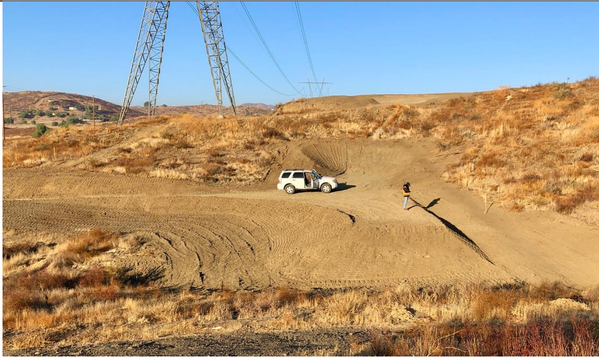
Photo 8 – The grading work for tower pad #130. Photo facing west
