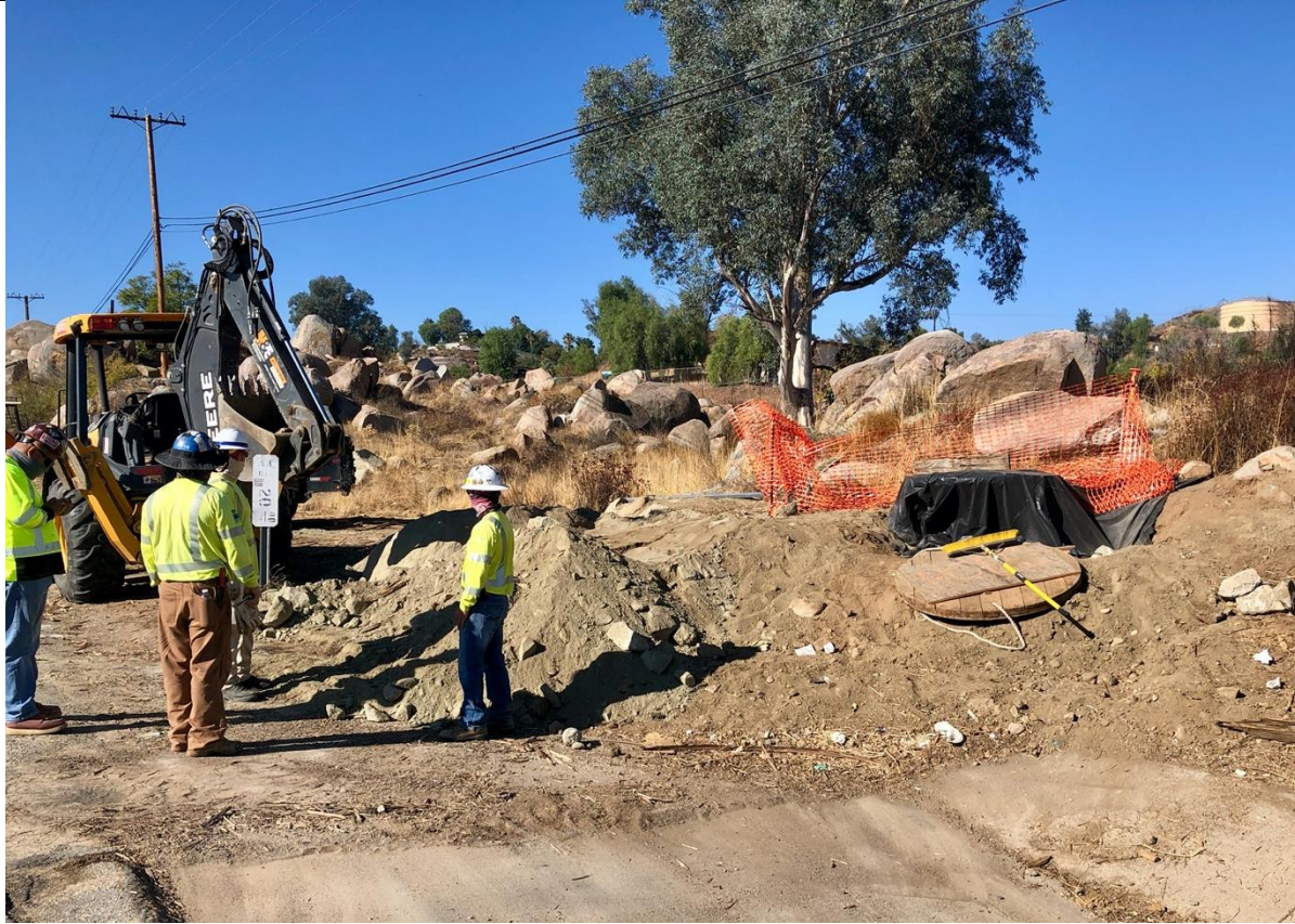
Photo 15 – Cleanup work at tower site 229 along Hwy 74. Photo facing west
