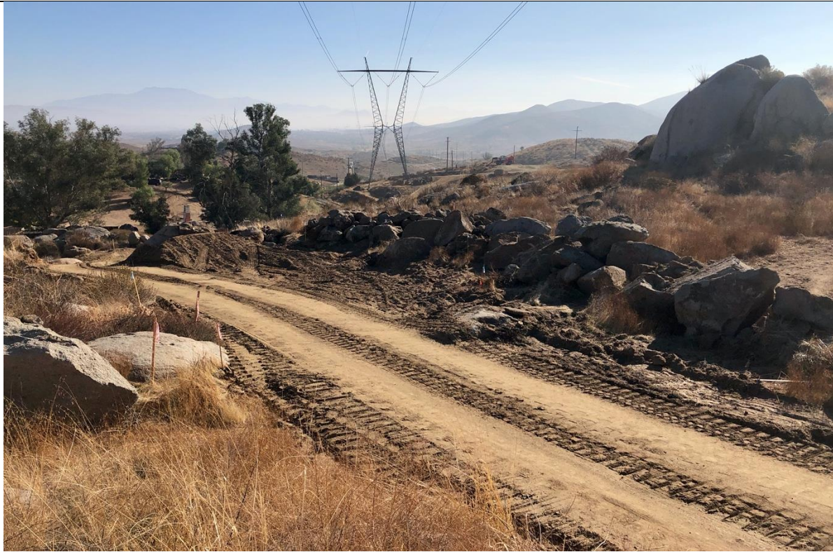
Photo 13 – Access road work between towers 144 and 145. Photo facing east
